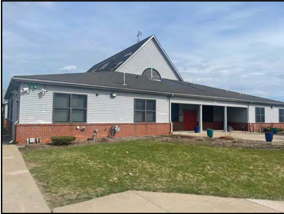
Photo 1: View of community building located at southwest portion of the subject property.
